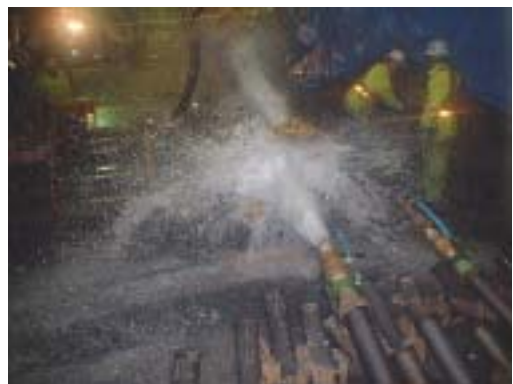
写真-1 湧水状況(2.1MPa, 5t/分)
